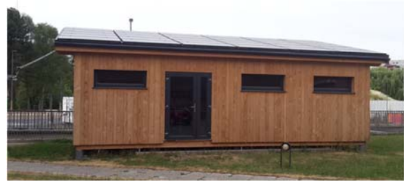
Fig. 9. SMART-EnR platform: photovoltaic chalet.
