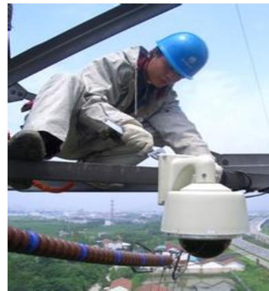
Fig. 1. Transmission lines danger point remote video monitoring system HD camera.
