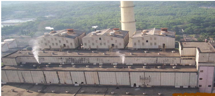
Fig. 6. Steam Generation Plant.
