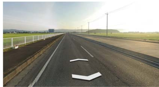
Fig. 19. Evaluation section view A very flat, two-lane bypass road with a central median running through the rural area.
